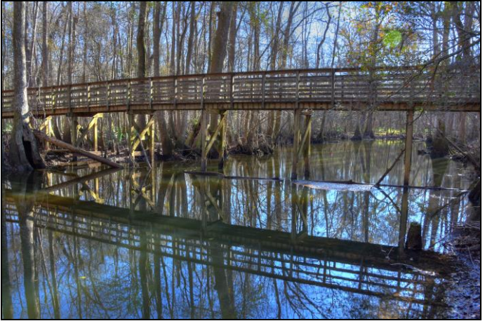
Rembert C. Dennis Bridge over Wadboo Creek on Palmetto Trail.
